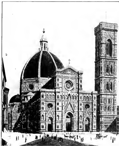
FAÇADE OF THE CATHEDRAL (S. MARIA DEL FIORE), FLORENCE Designed by Brunellesco
